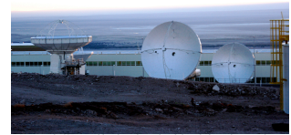
Antennas at the OSF received from the vendors, undergo holography for panel setting and pointing (left) before incorporation into the new science configuration (right) for final integration and verification. After this program they are transported to join the commissioning array at 5100m (far right).
